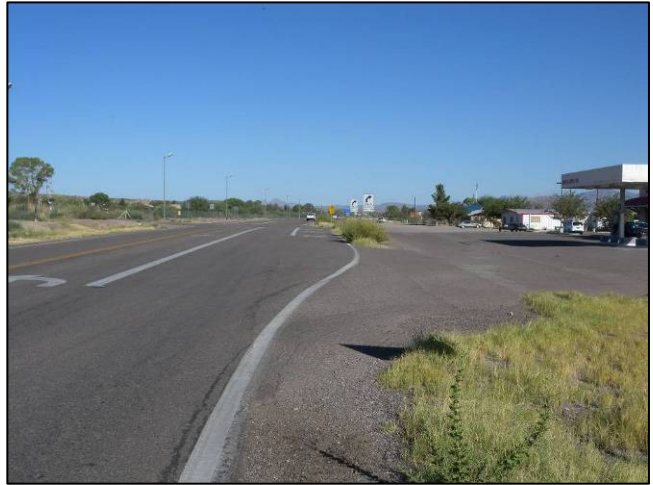
70-foot opening at Mt. Turnbull Market, located at the right-turn lane taper
